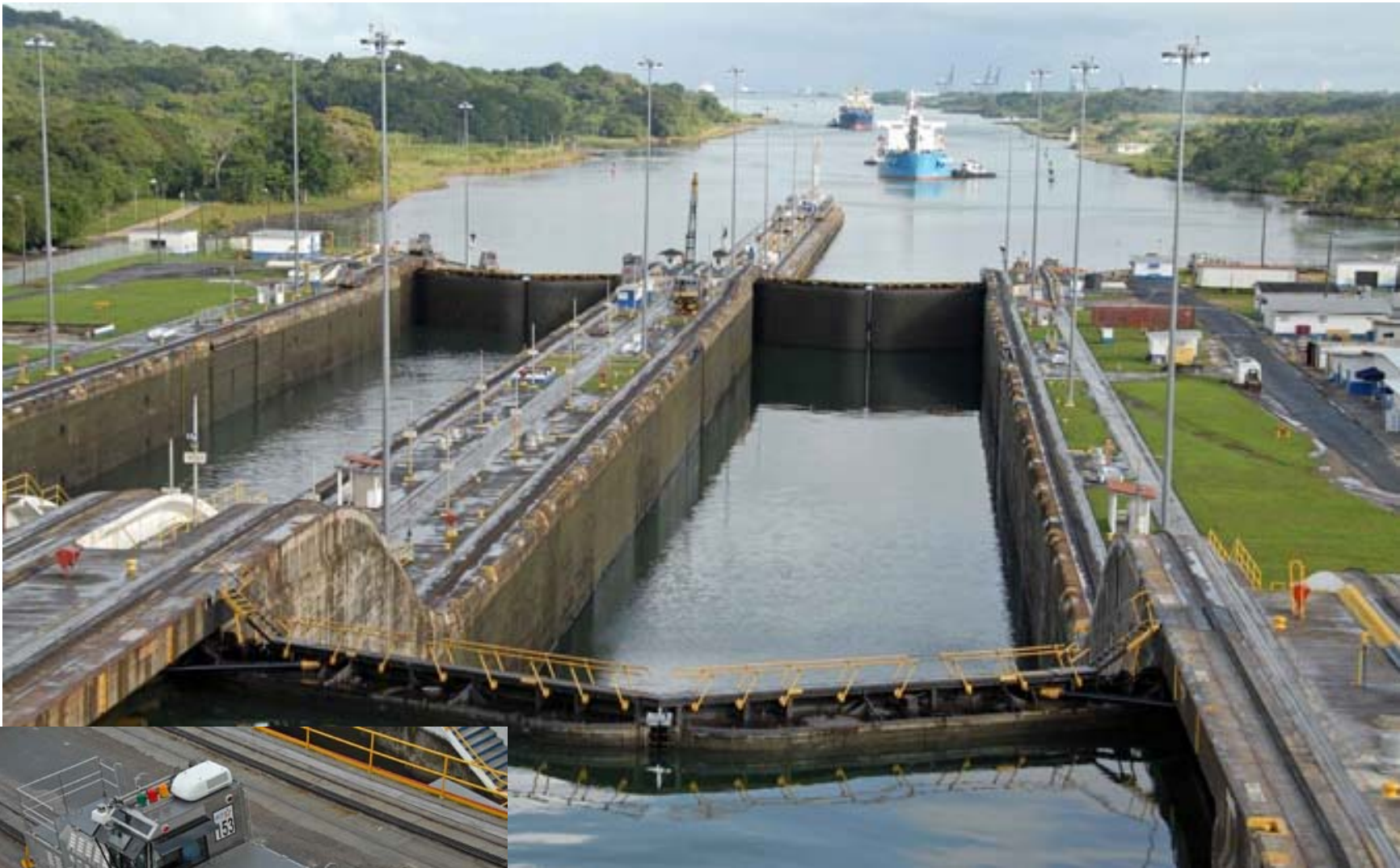
The gear driven locomotives (left) that are used to move the ships through the lock are called “mules”.
